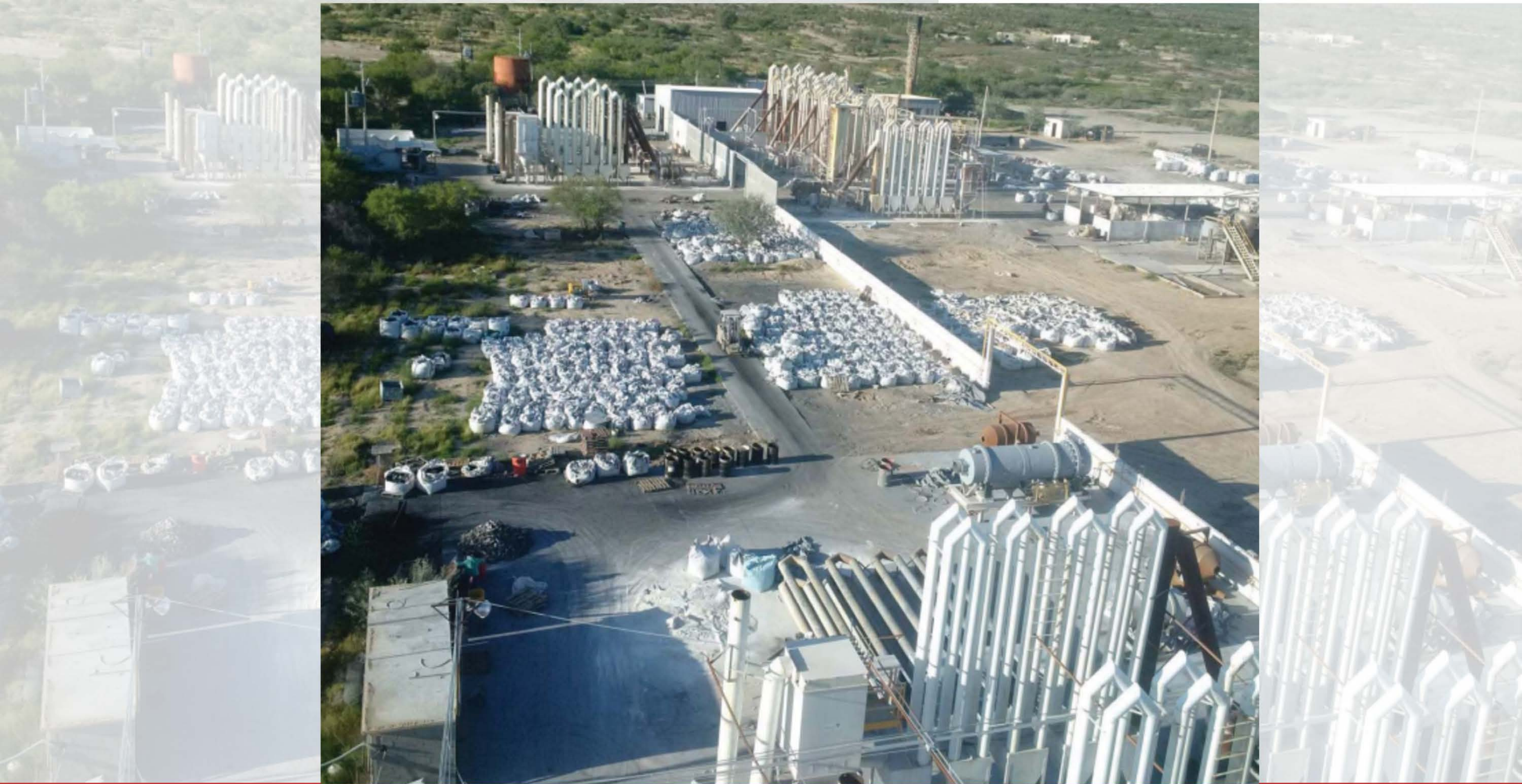
MADERO SMELTER PLANT - COAHUILA, MEXICO NOTE: SMELTER CAPACITY OF 200 TONS PER MONTH OR 7 TONS PER DAY
